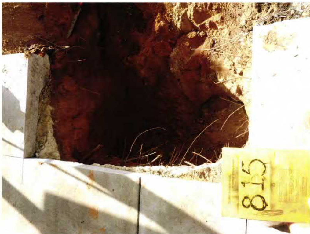
Picture 2: UST 815Azalea excavation.
